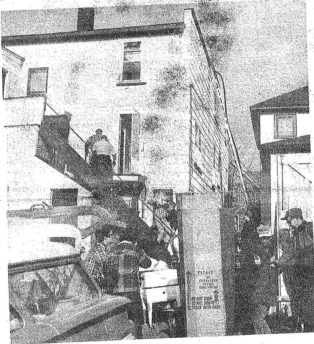
EVACUATION--four apartments in the Doherty Grocery building on Liberty-st. were evacuated while firemen stopped the third floor fire from spreading. There was considerable smoke and water damage. Before fire was controlled, neighbors, friends and residents carried out belongings. (NEWS photo by Fred Lovelace.)
