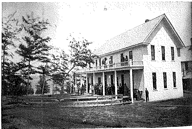
The Original Bay View House
