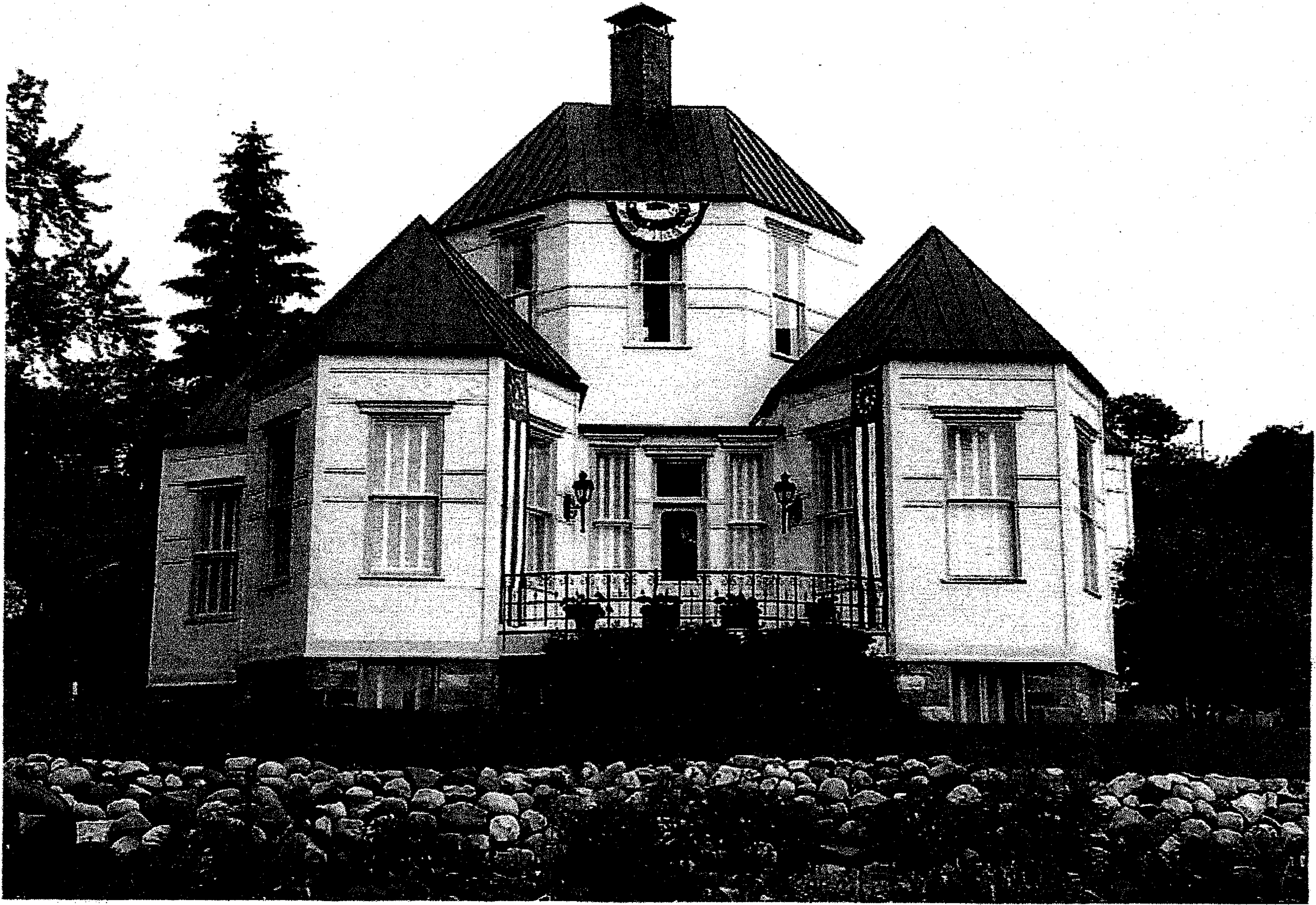
Ephraim Shay designed and built this hexagonal shaped house with six wings opening off the central core with a tower on top. The interior and exterior walls were stamped steel. It is still in existence at 396 East Main Street, Harbor Springs, Michigan.
