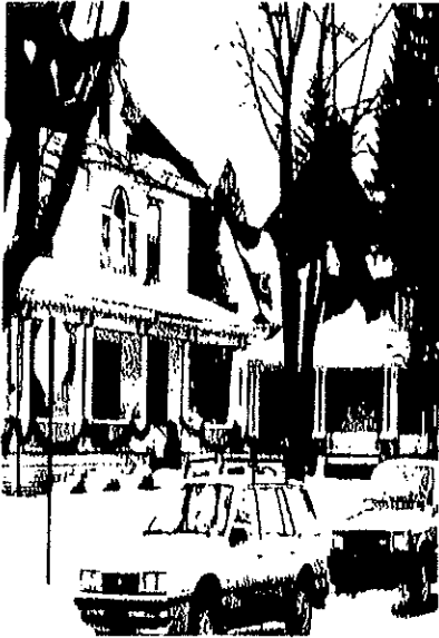
HOMES ALONG Mitchell Street are included in the East Mitchell historic district.
